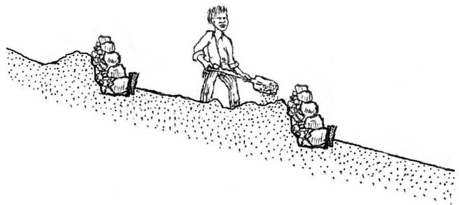
6. Use an A-frame and a rake to get the soil level. You will now have two terrace walls and a level terrace of soil between the walls. The final soil surface must be at least 10 cm lower than the terrace wall so that erosion does not take place.
