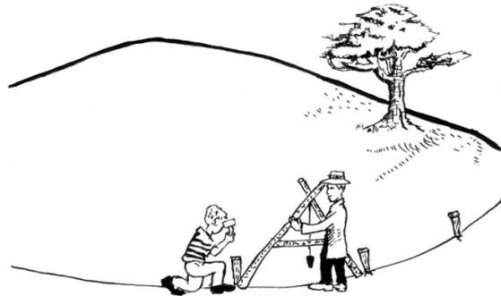
2. Dig a trench about 40 cm deep and 60 cm wide along the first contour line (see Table 1). Place the soil upslope of the trench.
