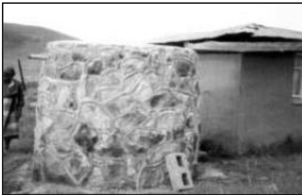
An example of a tank built from stone and cement
